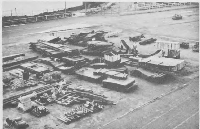
SECTIONS OF duct work, fabricated in halves in Japan, were lifted in bunches and placed on the pier. The dockside activity at No. 2 Finger Pier lends interesting patterns. SECCIONNAN DI tubo, fabricá na mitar pida na Japon, tabata worde hizá den grupo y depositá ariba waf.
